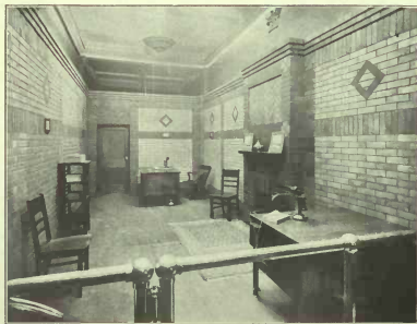
Show Room in Toronto Office, 50 Adelaide Street W. The walls of this room consist of eleven solid brick panels, each panel representing a different grade of brick.
