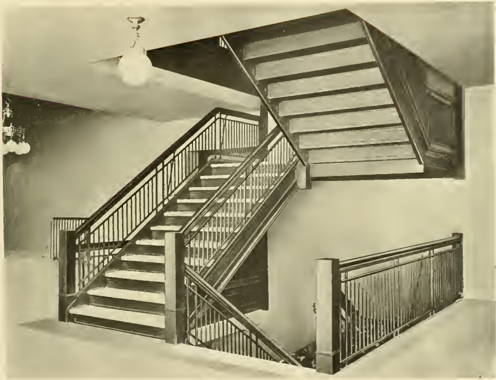
Cast Iron and Steel Stairs
