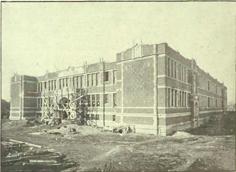
NEW MEMORIAL SCHOOL IN COURSE OF ERECTION AT HAMILTON
