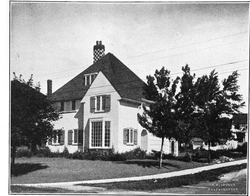
House of C. A. G. Matthews, Esq., Lawrence Park, Toronto. Murray Brown, A.R.I.B.A., Architect
