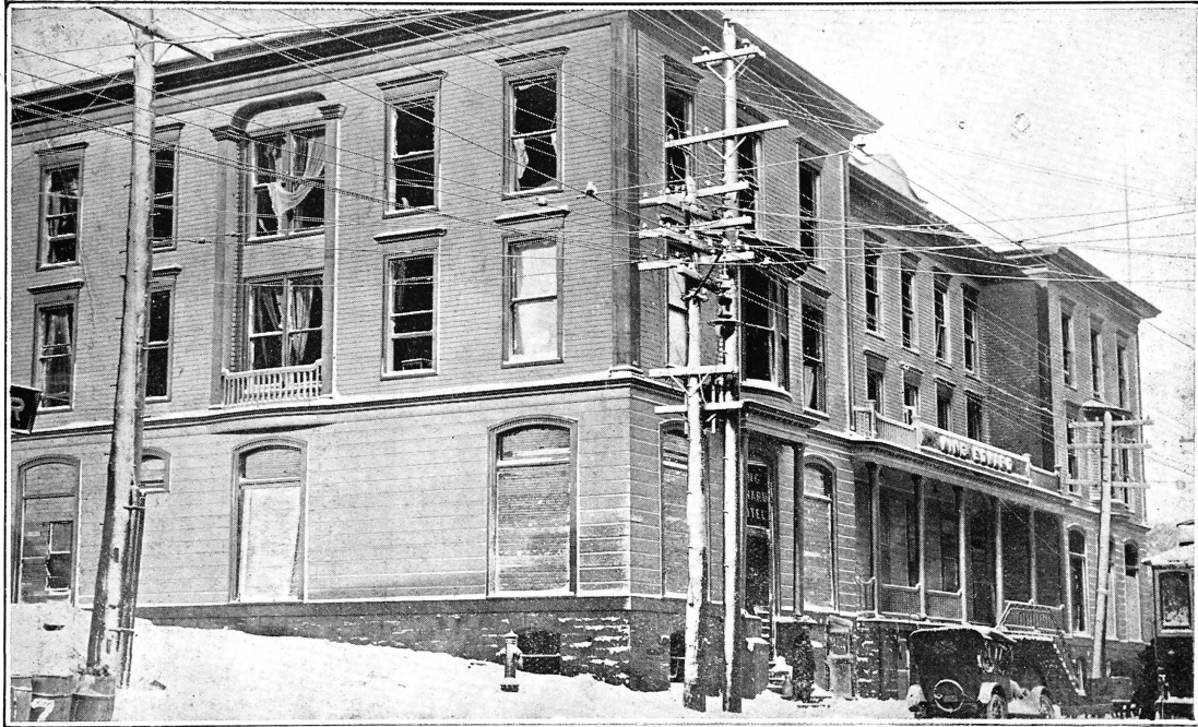
King Edward Hotel—opposite North Street Station. An employee in dining room was killed by flying glass. Photo by MacLaughlan
