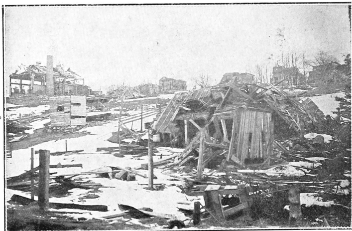
Desolation in Dartmouth. —A few of the many residences destroyed.
