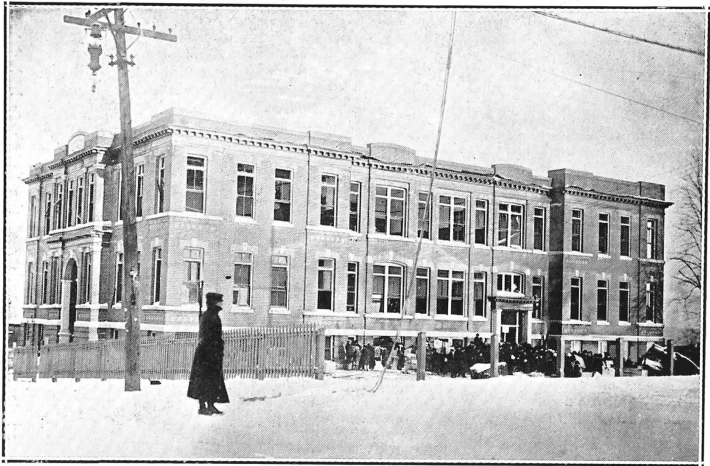
Alexander McKaye School. —Though badly damaged, it was used as a relief depot, where food was supplied to sufferers.
