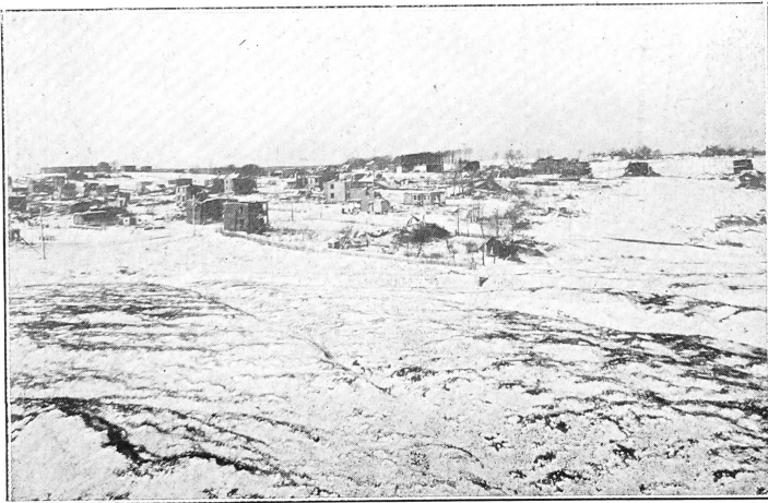
View from Fort Needham, showing general desolation of vast area over a mile from the explosion.
