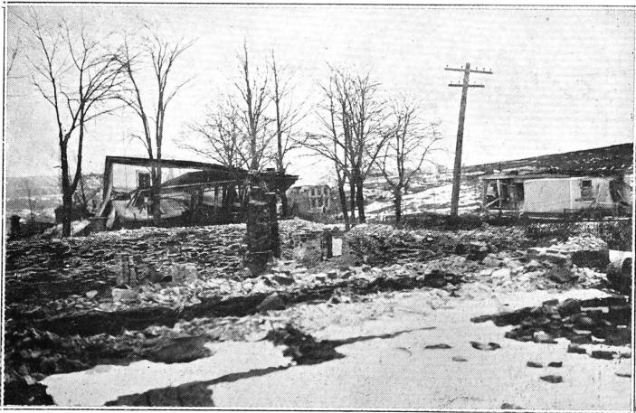
Gottingen Street. —Of many beautiful residences only destroyed foundations now remain.
