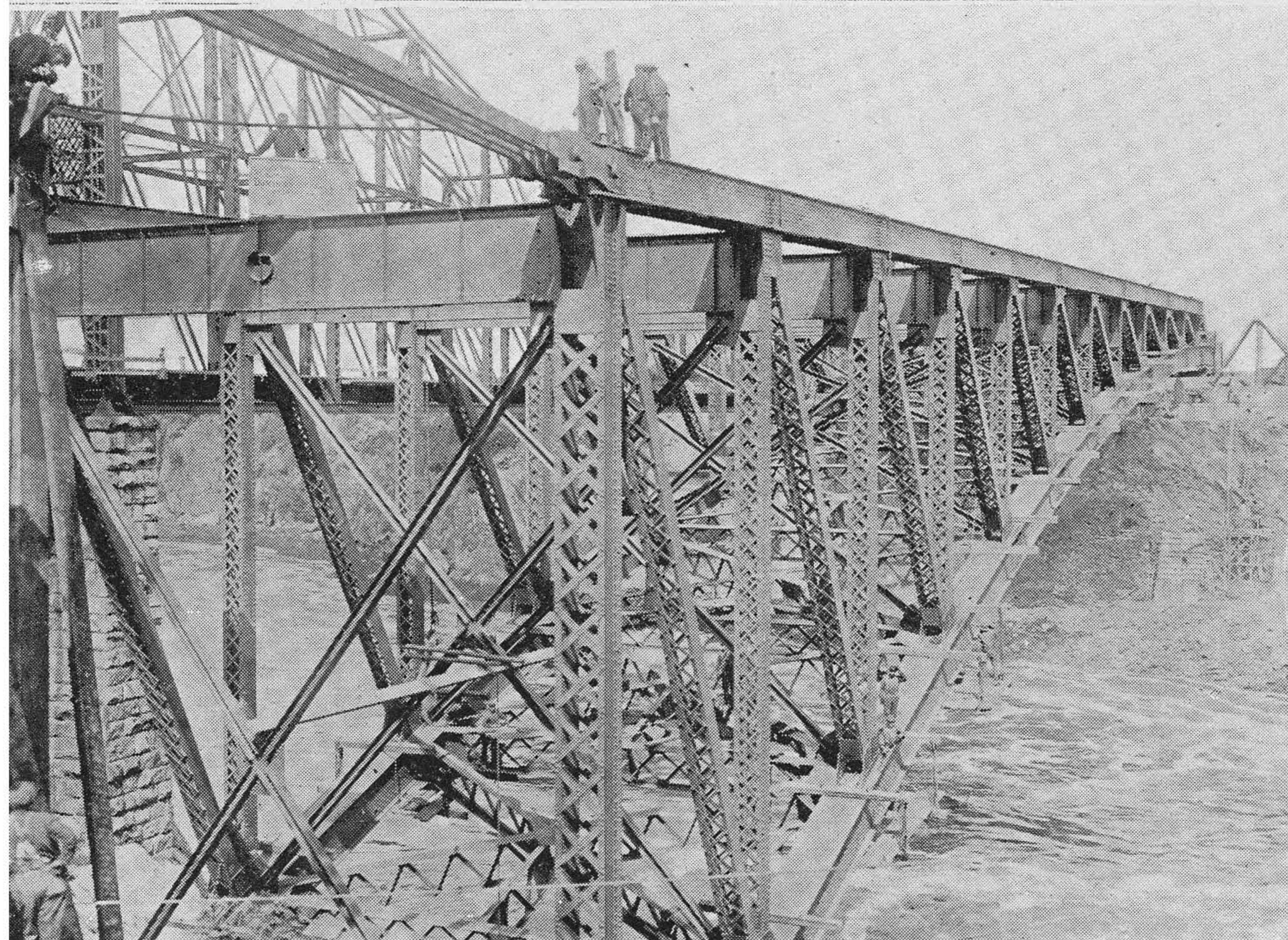
West end anchor bars. West arm cantilevered.
