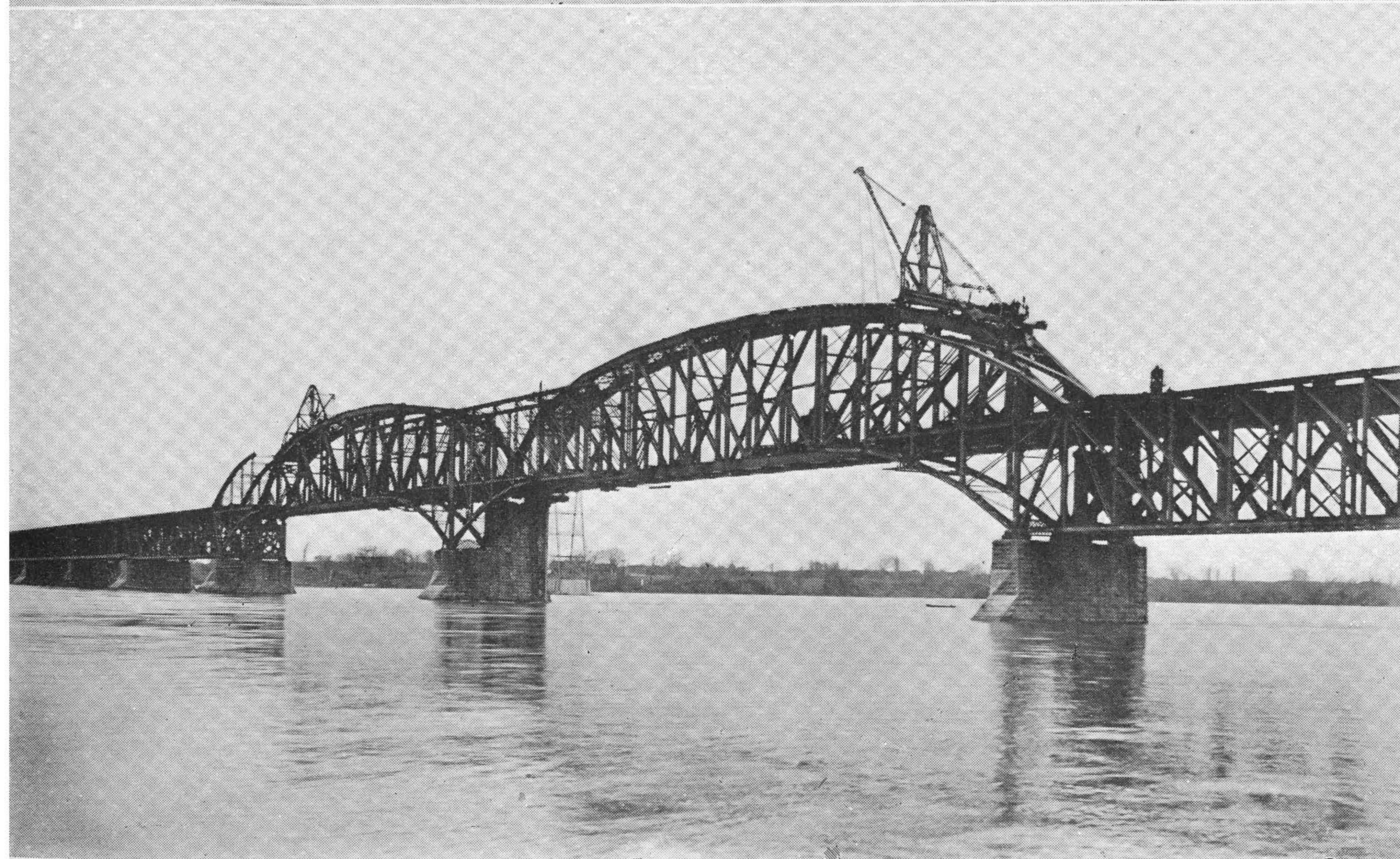
1st and 2nd 408 feet spans ready to launch Dismantling old channel spans
