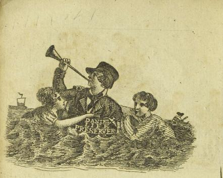
Mr. Daniel's Life Preserver, as exhibited passing through London Bridge. I have not time to describe the whole contrivance: but by means of a leather apparatus, which is put over the head, and buckled on, and which the wearer may fill full of air, a person may float, with ease and safety, for any length of time; and should the plan be generally adopted, it will doubtless be the means (as indeed it has already been) of saving many a valuable life\*.
