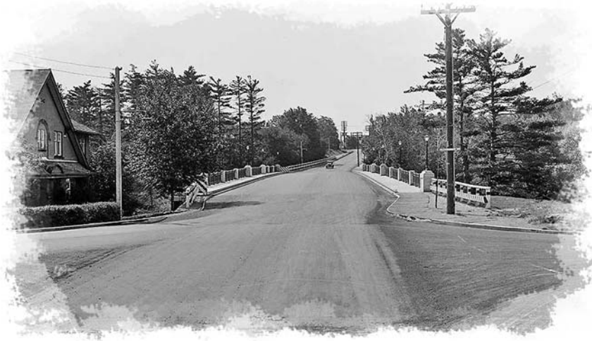
Mount Pleasant Bridge, looking south from Glengowan Road, 28 July 1936
