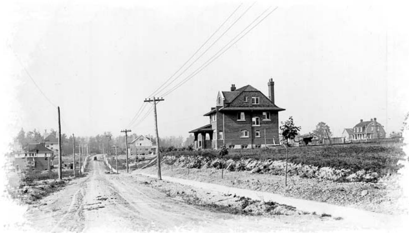
Dawlish Avenue looking west to Mount Pleasant Road, c.1914. 110 Dawlish Avenue is in the foreground.
