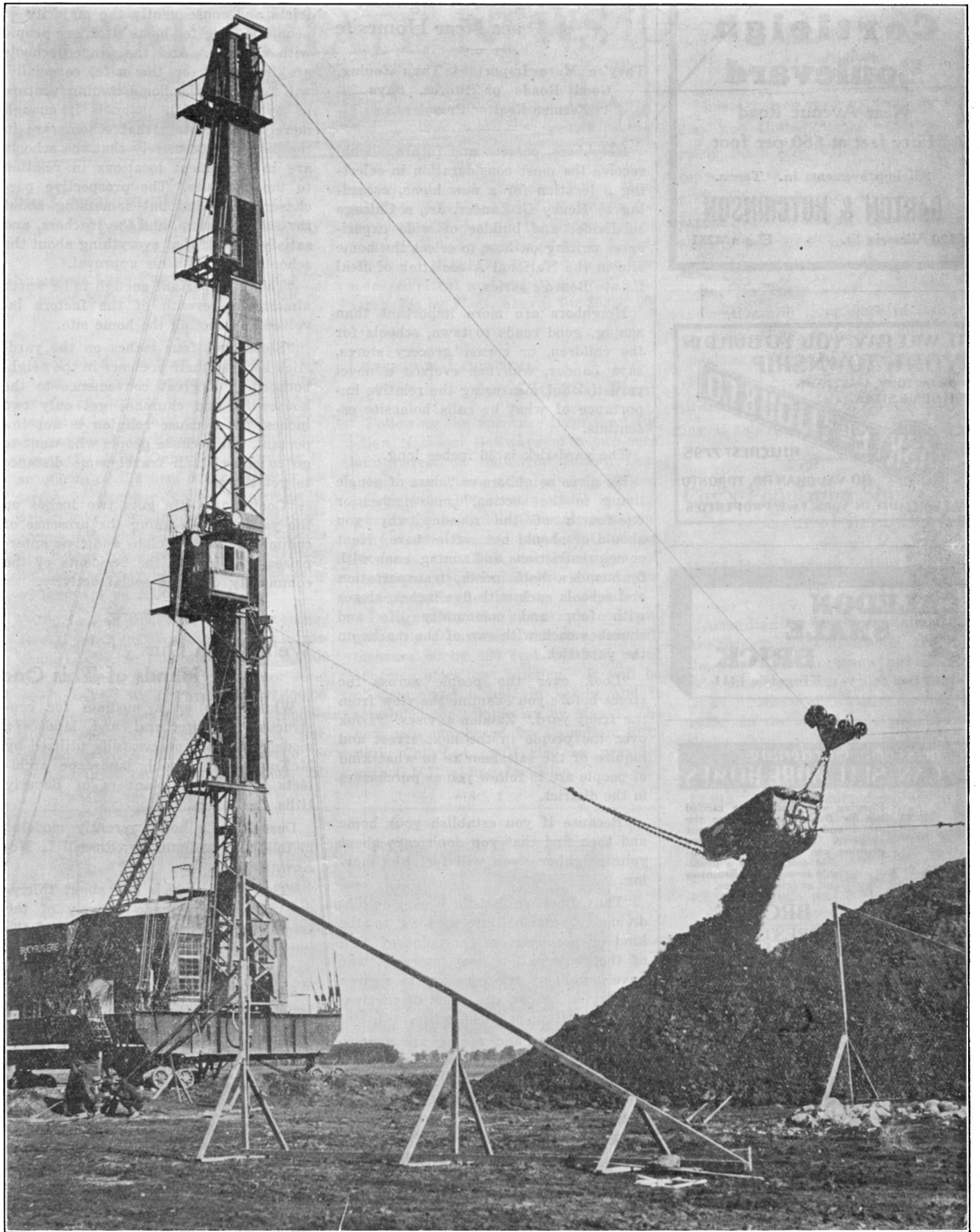
A mechanical giant at work at Beauharnois. One of the four steel tower excavators—135 feet in height—specially designed to dyke the route of the new Beauharnois Canal. It is operated electrically and its bucket handles 10 cubic yards of material at each swoop.
