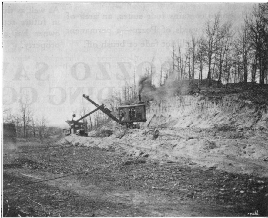
Work commenced last Monday on the extension of Wilmot Avenue from Weatherall Avenue to Bloor Street, east of Mossom Road. Here we see a steam shovel at work on the removal of a portion of the 31,500 cubic yards of earth, which will permit the opening up of 2,000 feet of frontage here. R. Home Smith & Company, Old Mill, are owners of this property and it will be offered for sale when this work is completed at the end of this month.
