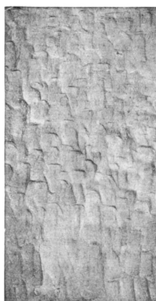
MOORISH A surface tooled promiscuously with the rounded corner trowel
