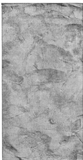
SPANISH A wavy, trowel-marked finish, smoothly irregular
