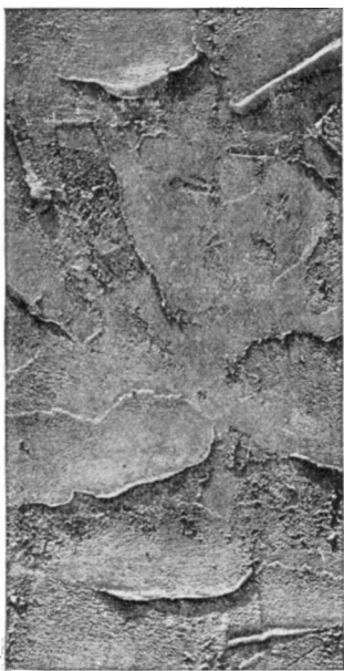
ENGLISH The irregularities are produced by side strokes of the trowel
