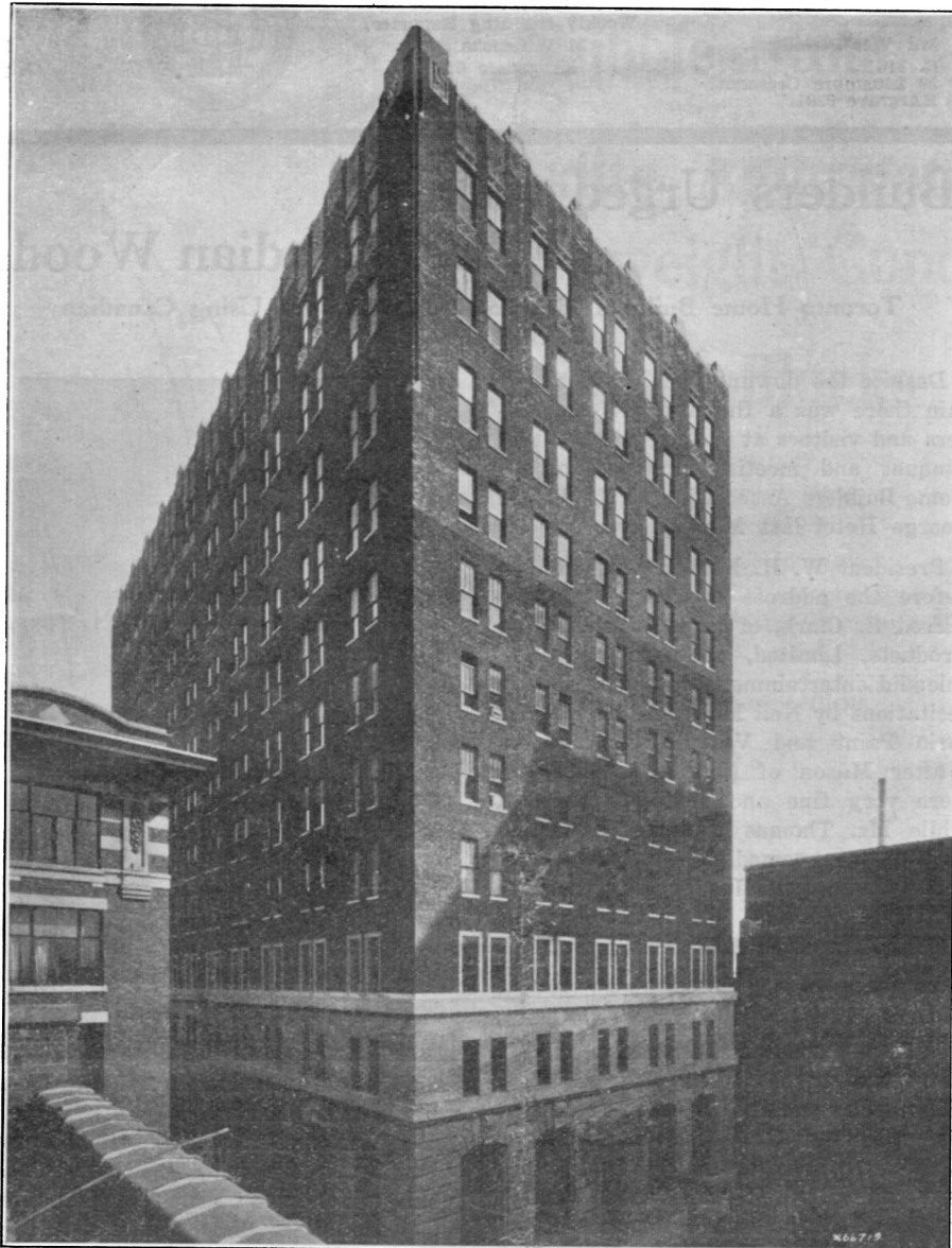
This imposing structure is the new Elgin Exchange Building of the Bell Telephone Company, situated at the corner of Adelaide and Sheppard Streets. The design has been provided by Chapman and Oxley, architects, 372 Bay Street, while the general contract was held and executed by Angus Robertson Ontario, Limited, 159 Bay Street. The entire building is faced with a special red range rough texture brick, backed up with Heath Load-bearing Wall Tile, both manufactured by Milton Brick Limited, 1158 Bay St., Toronto.
