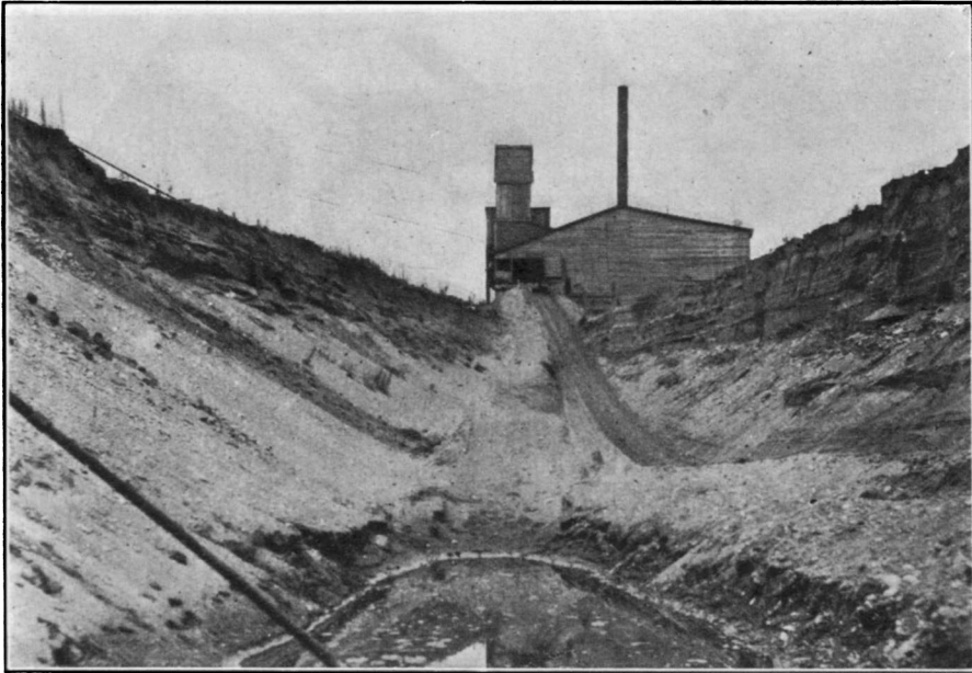
This photograph, taken from the bottom of the Perry Cement Company's gravel and sand pit, presents a rather unusual view of the plant, and also gives an excellent idea of the size of the pit. This material is conveyed into the plant by means of a drag-line. The path of the drag, or bucket, is plainly visible on the right, and the drag itself is seen just below the doorway through which it passes into the interior. The proximity of the pit to the plant effects a great saving in manufacture, in that the cost of hauling the material to the plant is at an absolute minimum.
