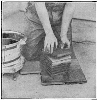
(1) Grasp block by opposite groove sides with both hands, face side of block up, tongue facing away from the operator. Fingers touch only the upper part of the grooved sides.
