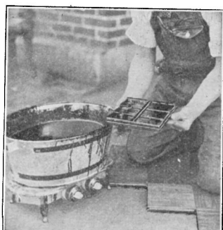
(4) Turn block into horizontal position bottom side up. This stops further draining and permits the adhering EVERBOND to flow evenly.
