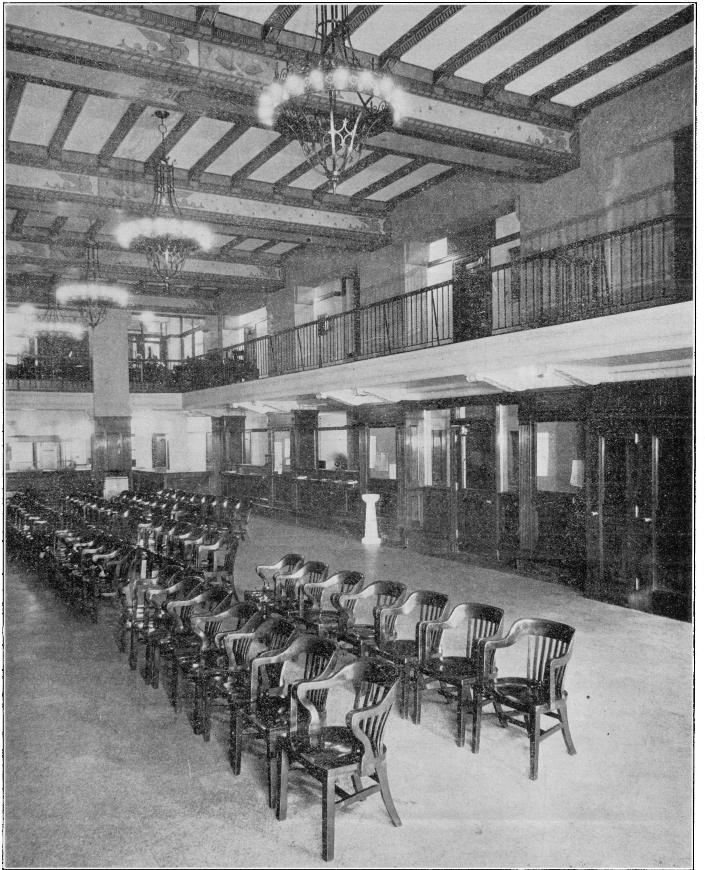
Board Room of Solloway Mills Building, showing panelling, counters and trim, etc., supplied by Rathbone.
