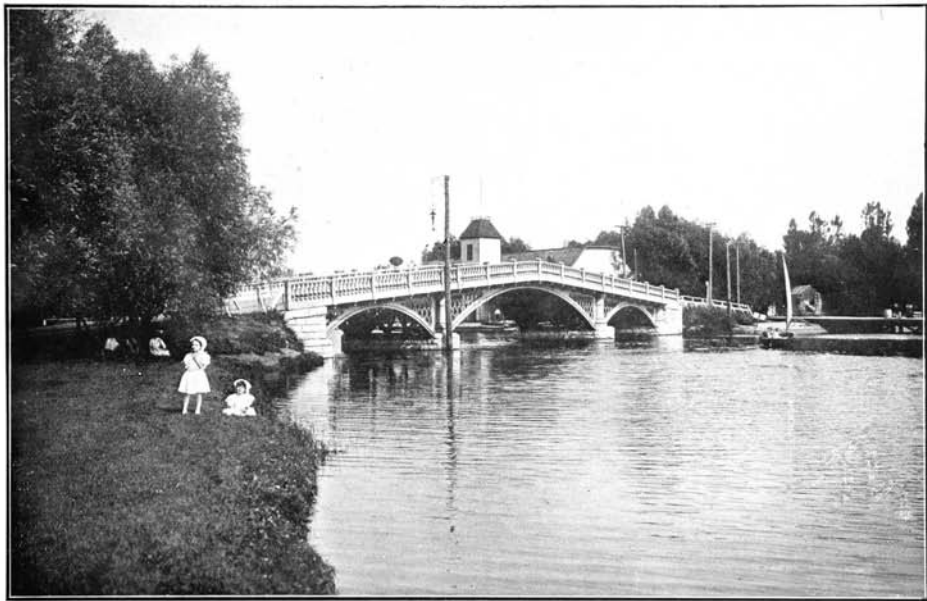
BRIDGE CROSSING LAGOON, Island Park.
