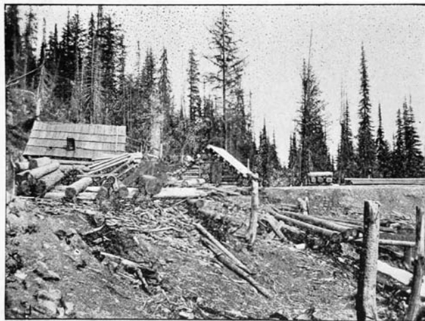
Wellington Mine, Whitewater.
