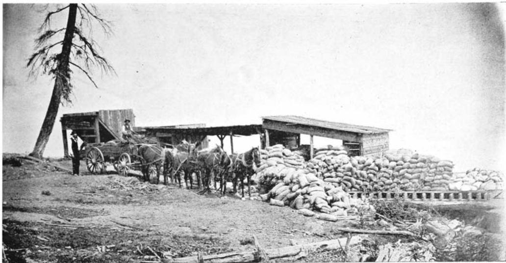
This is an exhibition of one of the famous shipments of ore from this district which has served to make it celebrated as a wealth-producer, second to none in the mining history of the world. It represents a shipment of one million pounds ready for transportation to the smelter from the Ainsworth wharf.
