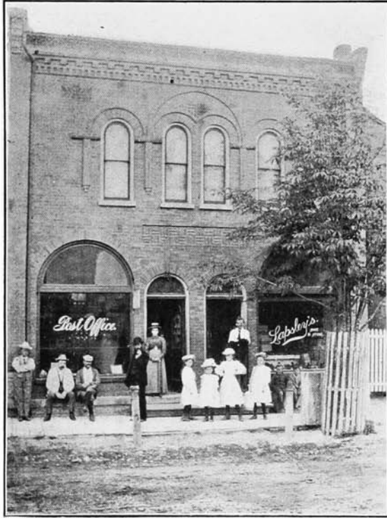
POST OFFICE BLOCK.
