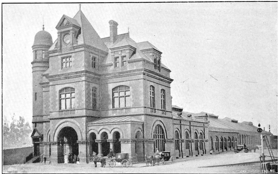
St. John Station on the Intercolonial Railway of Canada.
